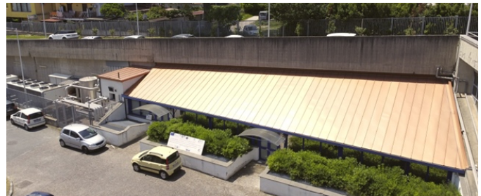
Fig. 1. The Data Center at Dept. of Physics
