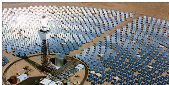
Fig. 9. Solar Two Power Plant (Wikimedia Commons License).
