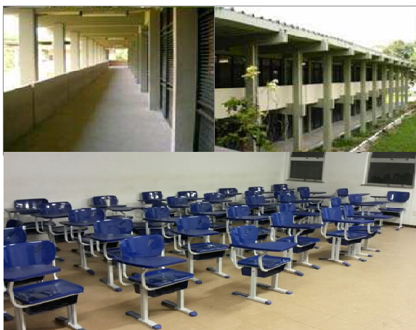
Figure 1. The classroom building: classrooms and side corridor
