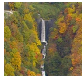
The reconstruction for one sub-frame missing
