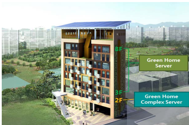
Figure 1 . Green home test-bed in KICT
