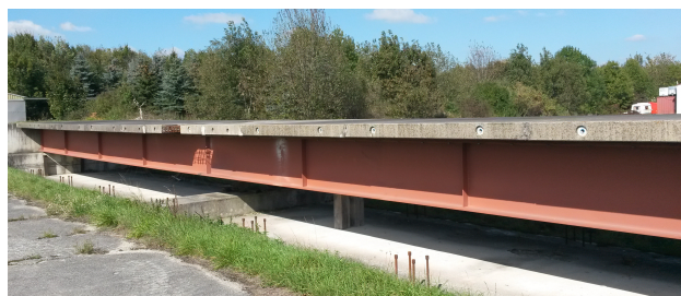
Fig. 13. The bridge for our experiment.
