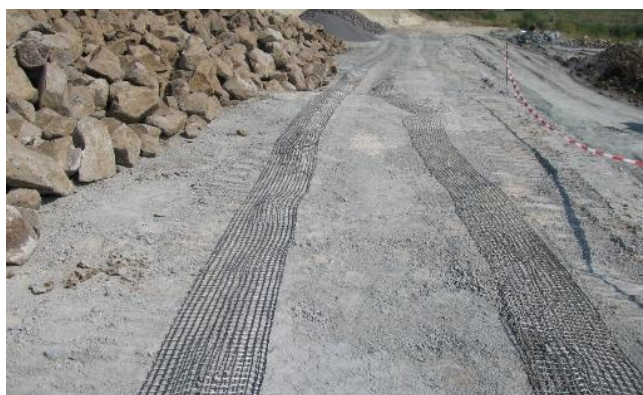
Figure 13. Geogrid with integrated fiber optical sensors.
